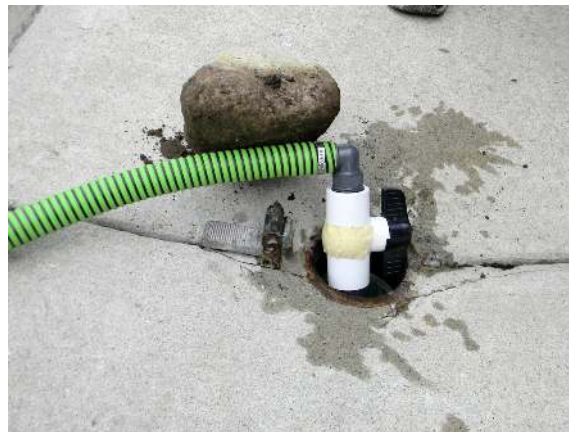
Use a convenient rock or other weight to hold hose down
