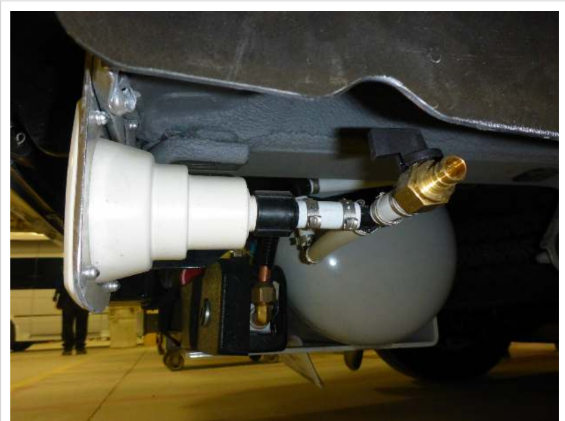
Rear drain behind the city water connection
