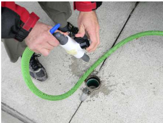
Open the valve on the end and insert into the drain
