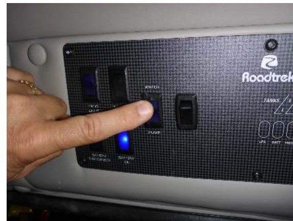
Water pump switch location on monitor panel
