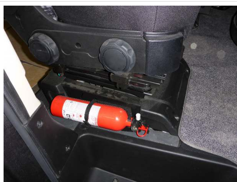
Fire extinguisher located at front passenger seat doorstep
