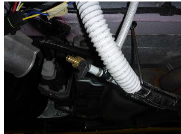
Fresh water tank drain, under driver's doorstep
